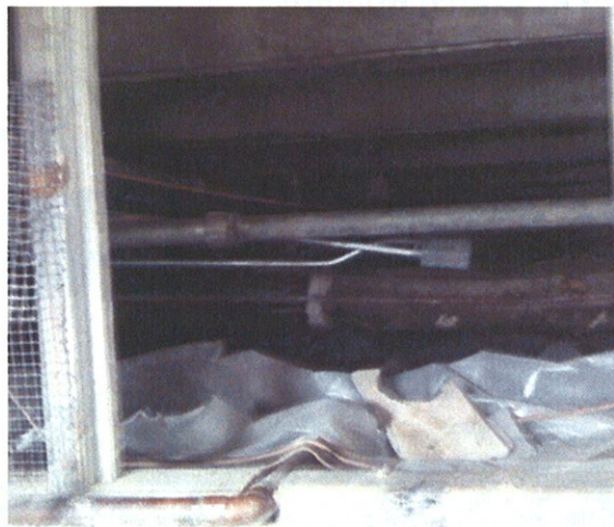
Old Pipes That Cause Major Flooding Problems
